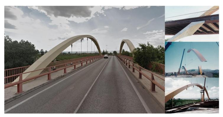
The bridge over the River Júcar comprises a double arch with an intermediate composite deck which is highly skewed.
